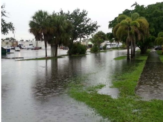
Impacted water managements systems
